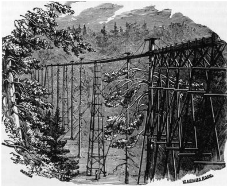
WATER FLUME ACROSS A HOLLOW BETWEEN RIDGES.
